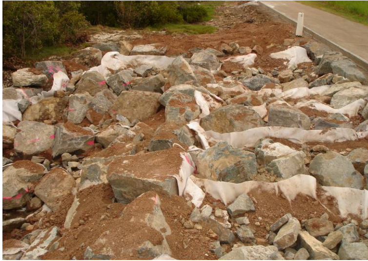
Figure 2. Construction of St Lawrence Fishway 1
