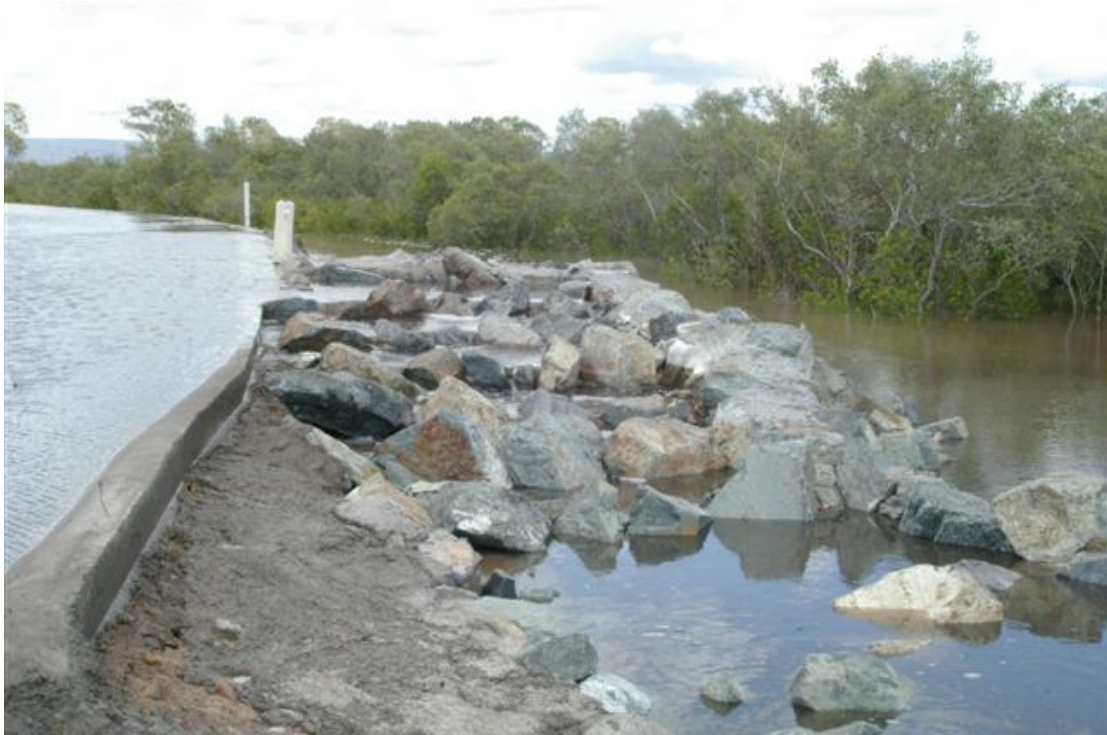
Figure 12. Rock ramp fishway constructed on the St Lawrence wetland.
