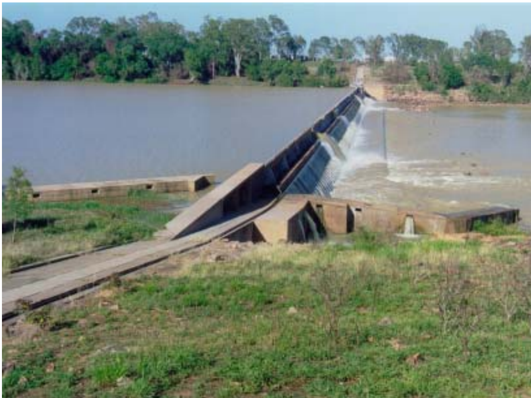
Figure 3. Clare Weir, focus of the current study. The existing ineffectual fishway extends from left to right against the bank in the foreground.
