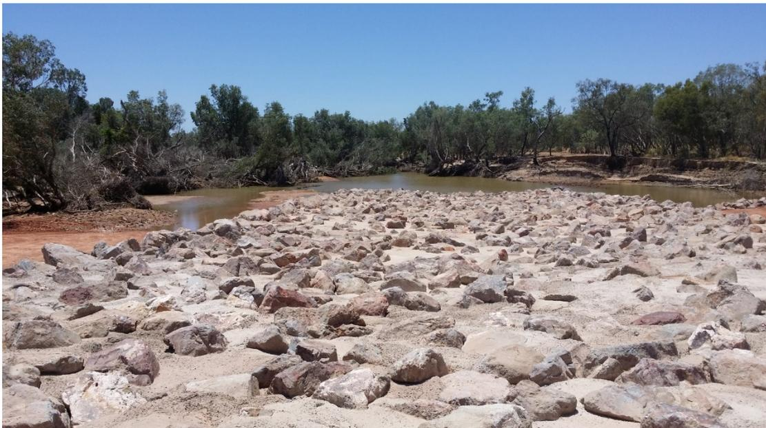
Figure 7. Secondary rock ramp fishway on the right abutment.
