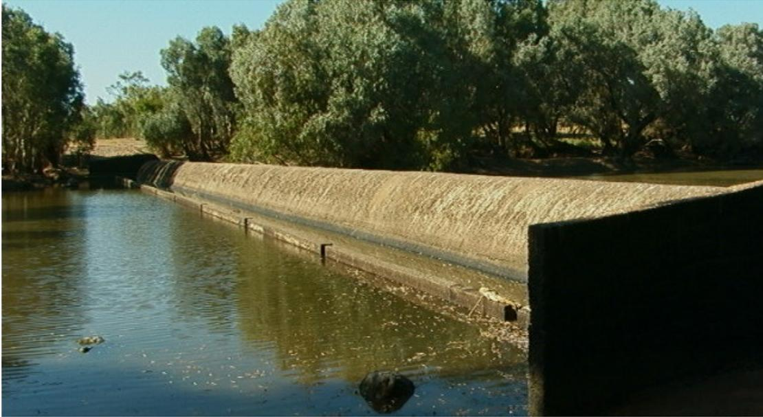
Figure 1. Glenore Weir prior to raising in 2016, wall height 2.18m.
