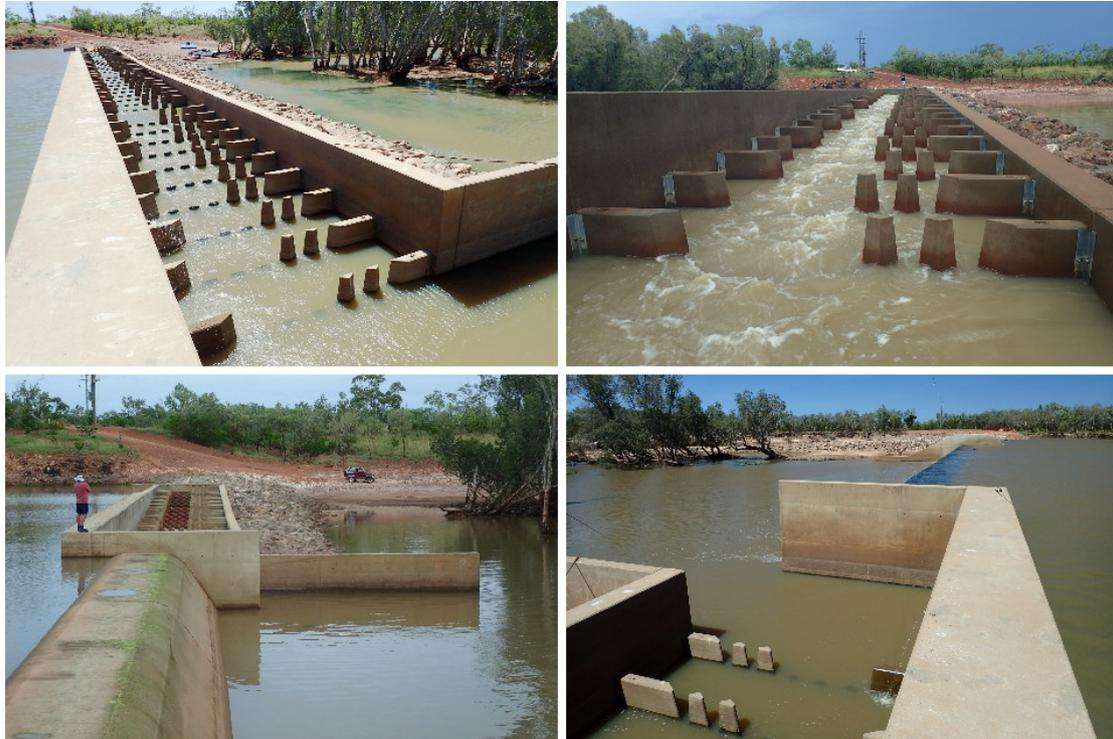
**Figure 2. Left bank side of Fitzroy River Barrage showing the fishway, Gate 1 and ogee crest structures. Image from Google Earth.**
