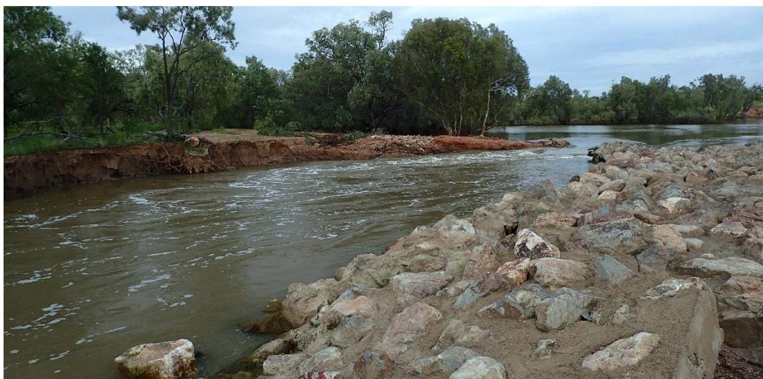
**Figure 18. Breach around the weir on the right abutment.**
