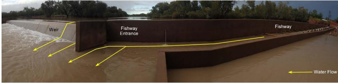
**Figure 19. Location of the fishway entrance adjacent to the spillway of the weir.**
