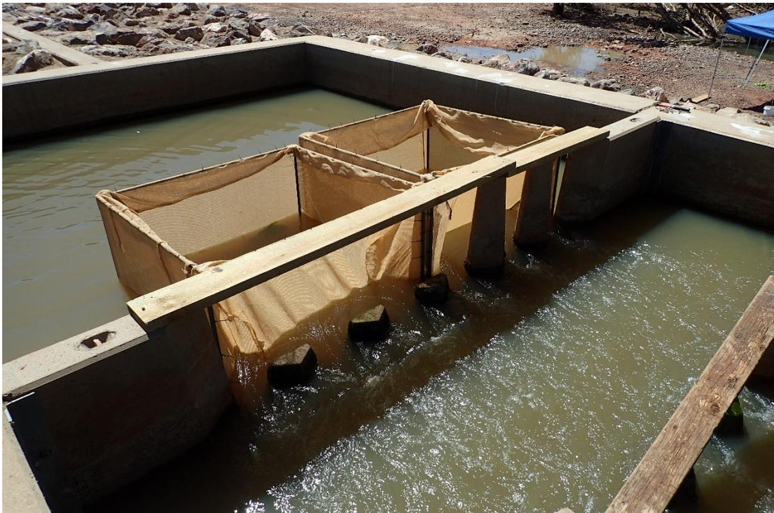
**Figure 3. Cone fishway traps located at the exit of the fishway during a top sample.**
