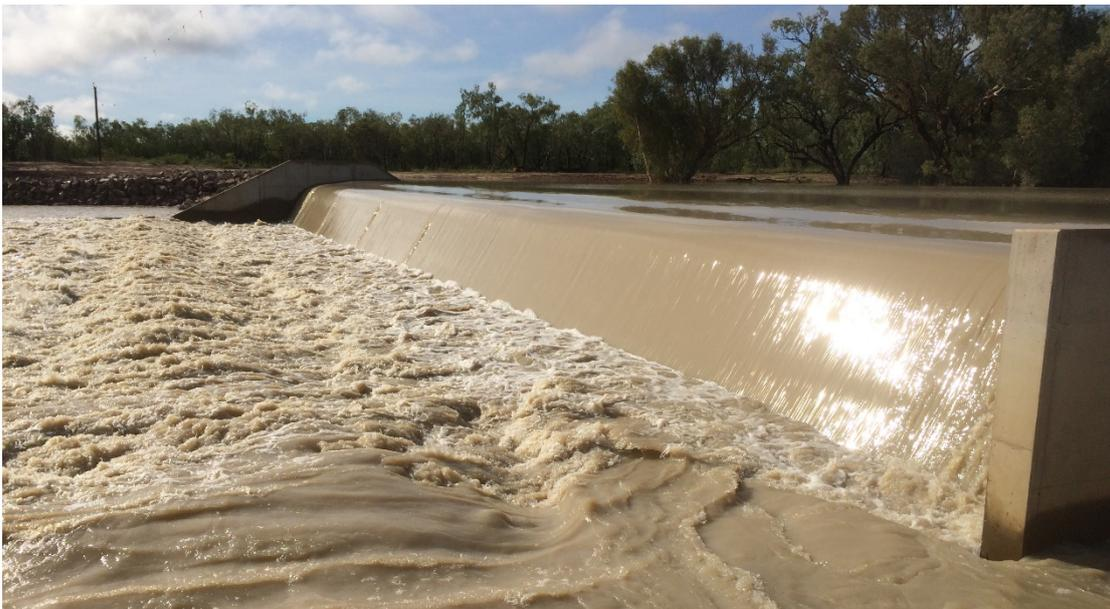
Figure 4. Glenore Weir after raising in 2016, wall height 3.68m
