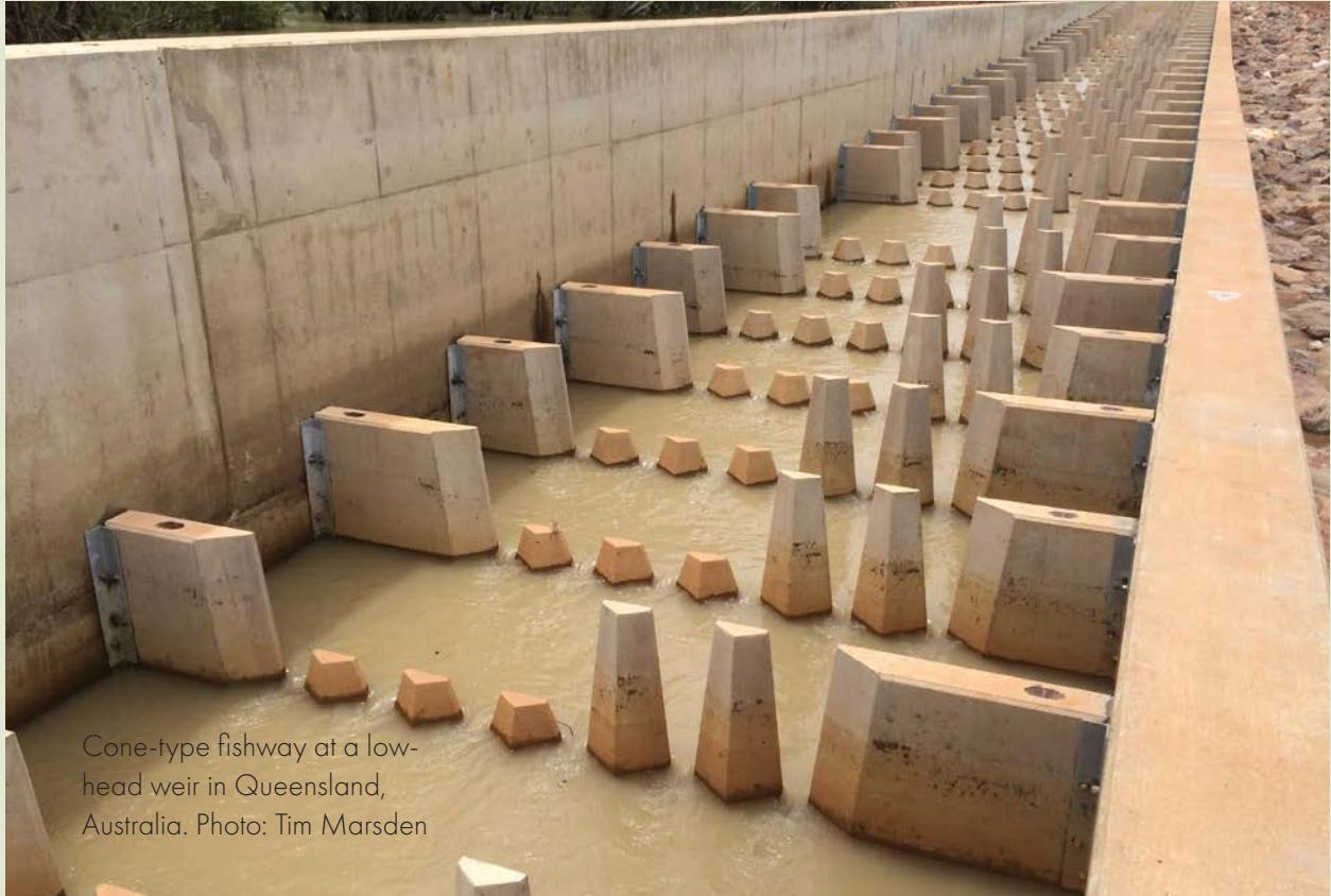
Cone-type fishway at a low-head weir in Queensland, Australia. Photo: Tim Marsden
